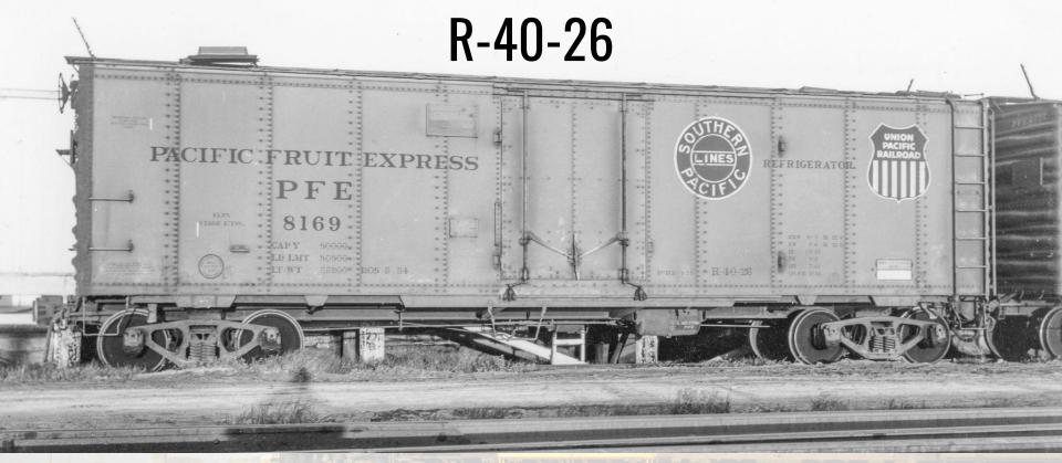
This excellent image with its low lighting highlights many of the details of the welded underframe. Note the updated paint and lettering with the lines dropped above and below the reporting marks.
