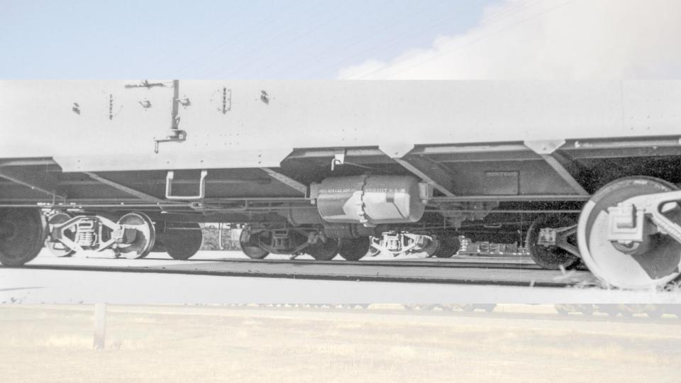
In 1941, Pacific Car & Foundry delivered 1,000 cars that were quite similar to the R-40-10, with several enhancements. The cars were placed in the series 44701-45700 and assigned to class R-40-14. Changes from the -10 class included round (W) corner Dreadnaught ends, Equipco integral hatch covers, convertible ice bunkers, plywood lining, and placard boards.
