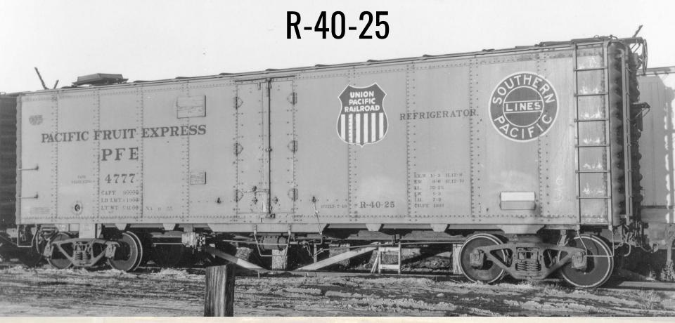
Once repainted, the side sill support "tabs" and the center sill step below the door opening were also the same color as the car side
