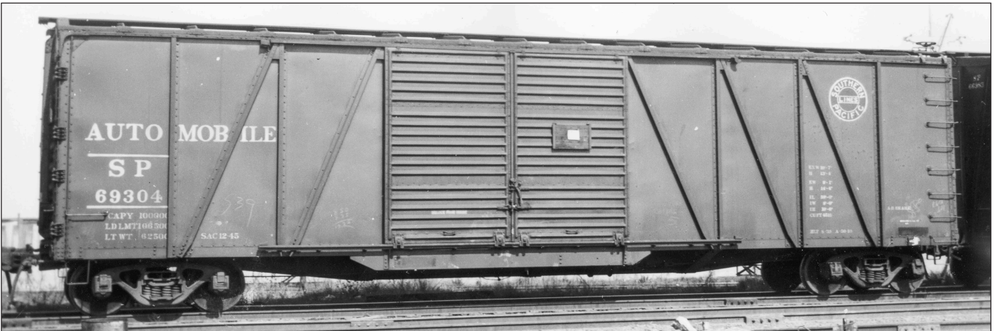
A-50-10 SP 69304 was photographed in Alameda (Oakland area) California in 1947. Note the hinges at the left corner of the car, for the Dreadnaught end doors. Howard Ameling Collection
