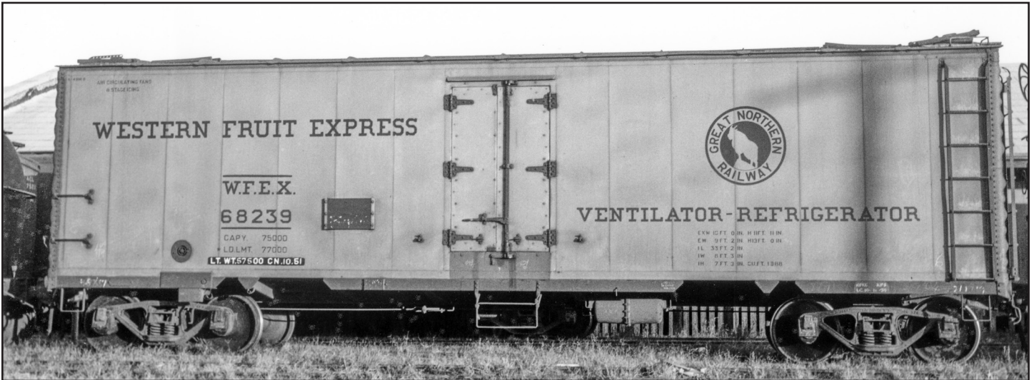
American Car & Foundry built 400 cars in 1948 that were nearly identical to the FGEX 38635-series. The cars were assigned to series WFEX 68000-68399. Notable differences from the FGEX cars included ASF A-3 Ride Control trucks and r+3/3 Improved Dreadnaught ends. The cars used Equipco integral ice hatches.
