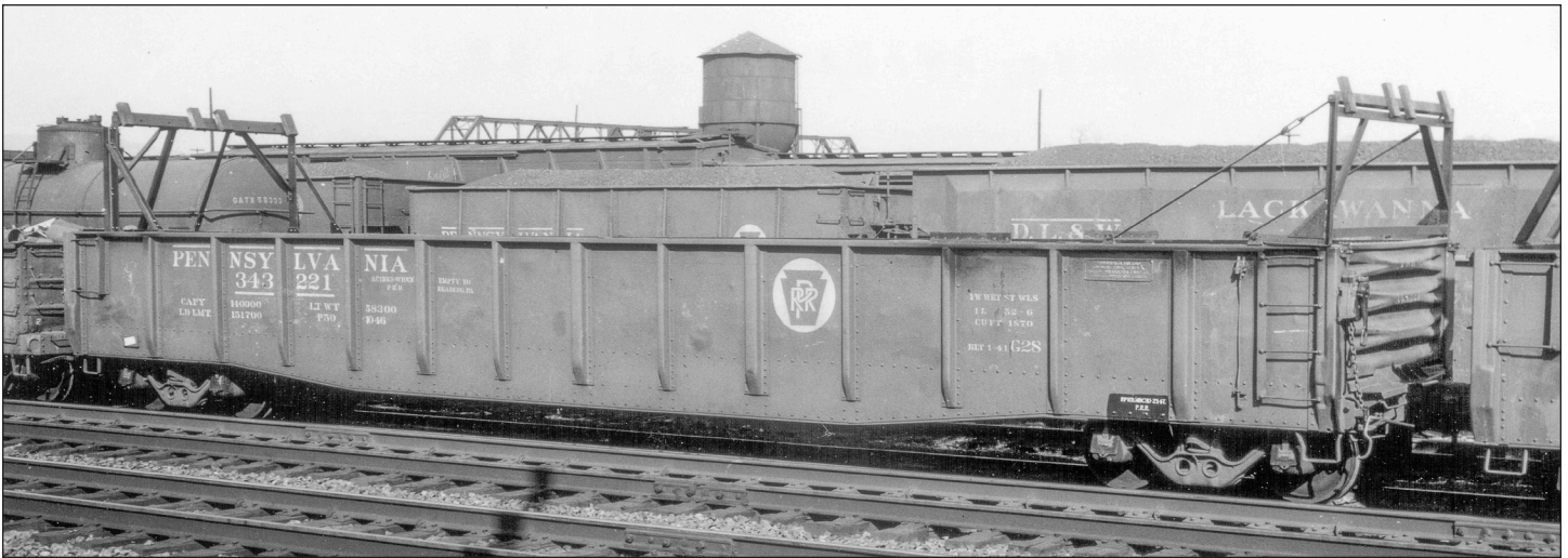
A G28 equipped with racks for transporting automobile frames. Bob Charles Collection, NMRA Kalmbach Memorial Library
